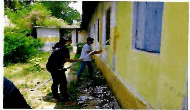
Exterior Wall Painting at Devi Vilasam School,
